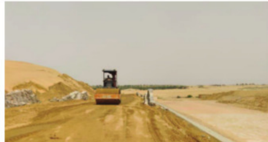
Work is underway on mega reservoir in Thar desert
